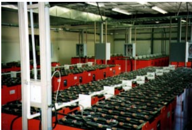
Fig. 2. 5600-kWh of C&D motive power batteries.
