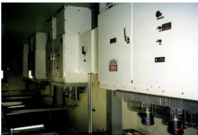
Fig. 3. Trace Technologies power processing system.
